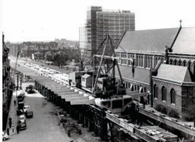
The Hammersmith Flyover under construction in 1960, cutting across the grounds of St Pauls Church.
