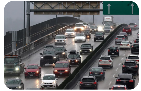
Second Narrows Bridge Traffic / Nick Procylo
